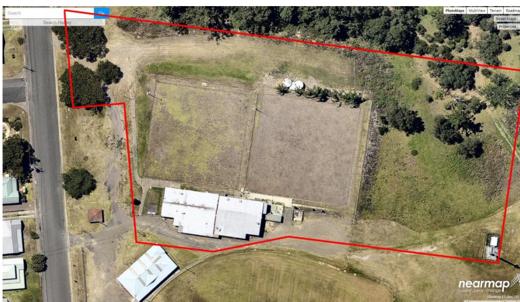
Figure 4. Location image; the subject land is outlined in red. The former clubhouse, bowling greens and associated infrastructure are visible. Note the variable nature of the vegetated and cleared areas of the site. Much of the site is set back from Edward Street on account of the Morpeth Common/sportsground car park and Hunter Water sewer pump station. Nearmap (by licence)
