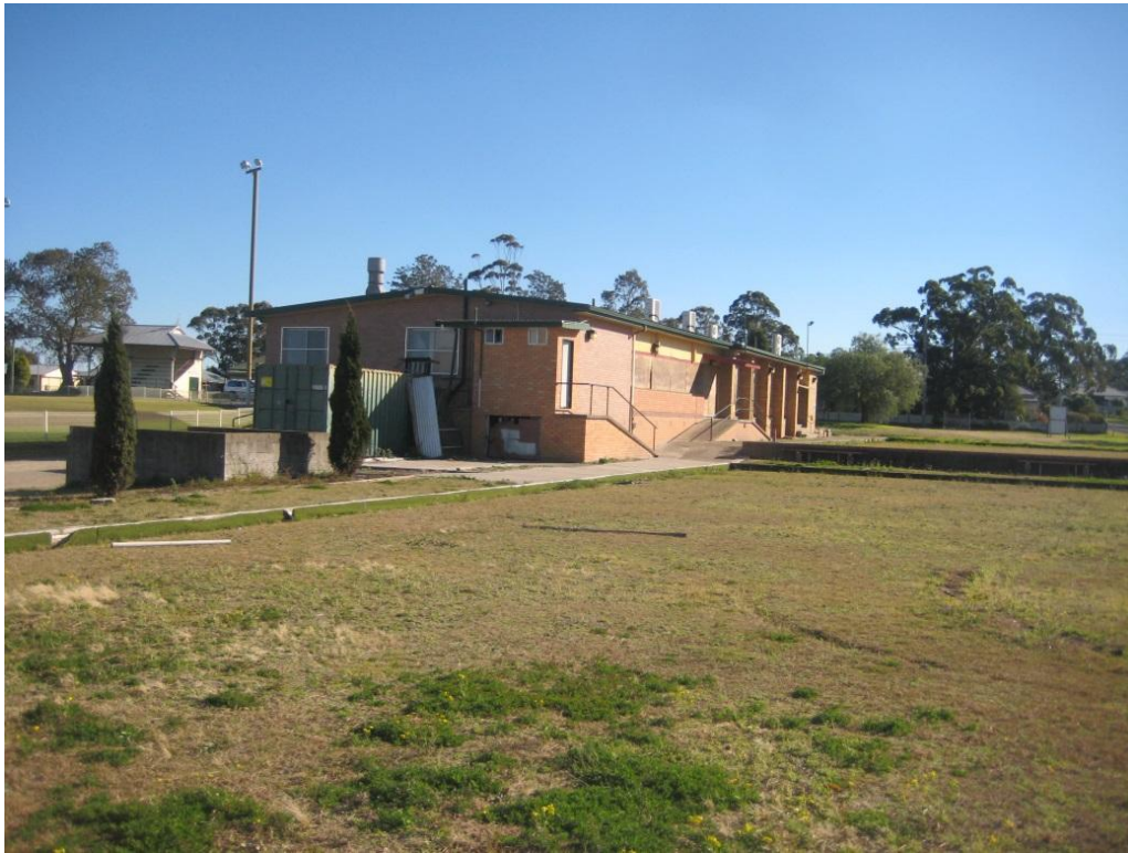
Figure 16. Former clubhouse, looking south-west, with grandstand in distance.
