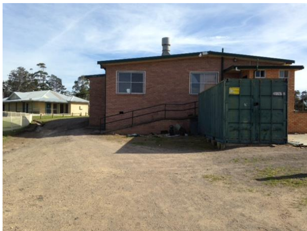
The informal car park located along the southern boundary adjoining the clubhouse
