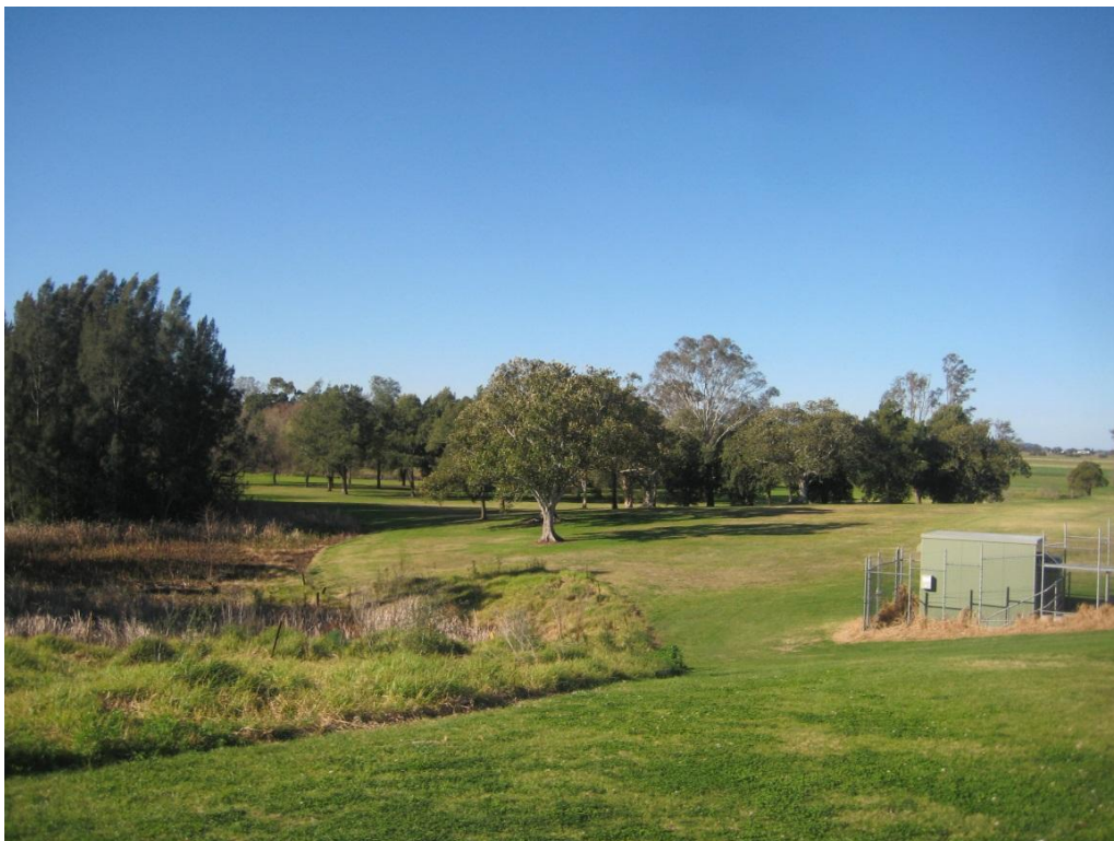
Figure 27. Looking south-east, showing Testra telephone tower enclosure at right.
